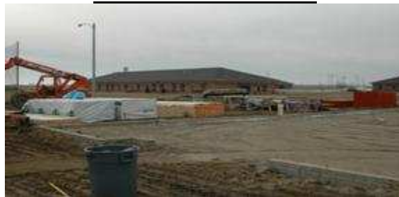
Construction material onsite at Jamani Java
